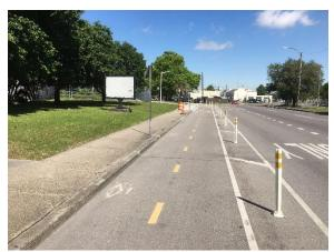
Figure 5. A cycle track with a striped buffer and delineator posts in New Orleans, Louisiana.
