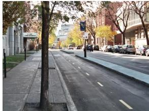
Figure 6. A cycle track with a concrete buffer in Montreal, Canada.
