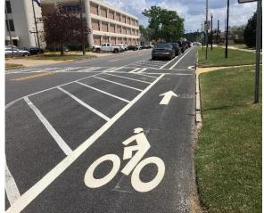
Figure 4. A bicycle lane buffered by striping and onstreet parking in Columbus, Georgia.
