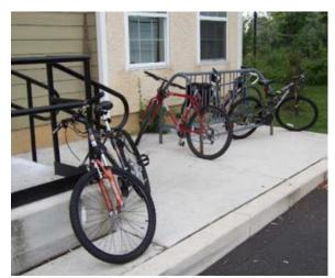
Figure 1. Older style of bicycle rack, colloquially known among cyclists as a "wheel bender." Note how bikes have been locked to the ends of the rack to avoid the wheel-bending effect, and one cyclist has avoided using the rack altogether. Source: First State Bikes
